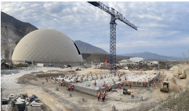
Concrete works at the flotation plant
