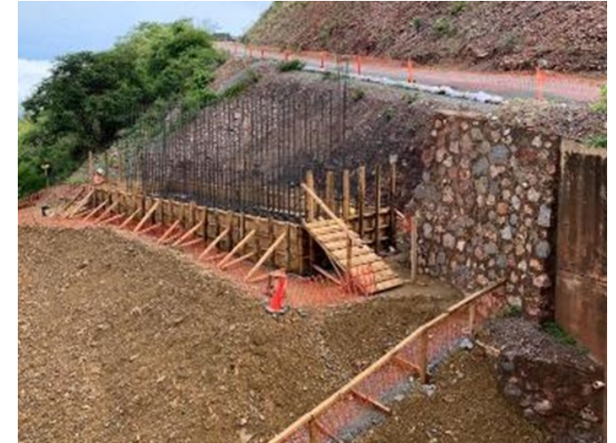
Pouring footing for Mazapa bridge
