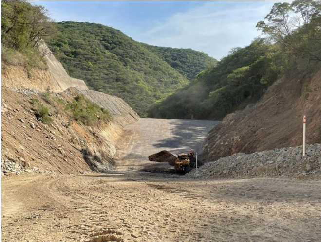
Sedimentation pond construction
