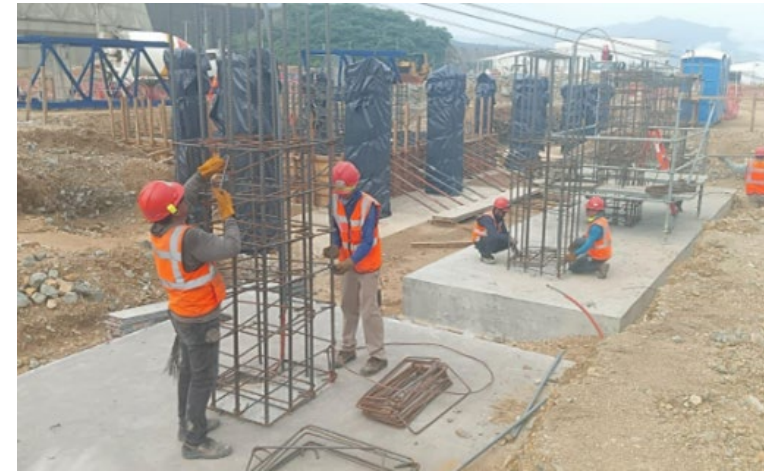
Footings for tower crane and flotation cells
