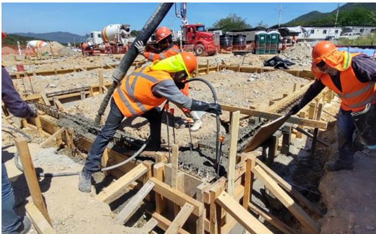
Pouring foundation for comedor at MML camp
