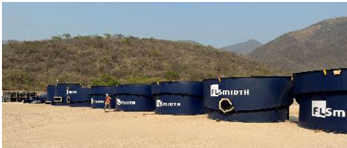
Copper flotation cells arrive at site
