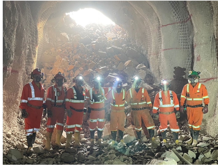
West Adit Vent breakthrough
