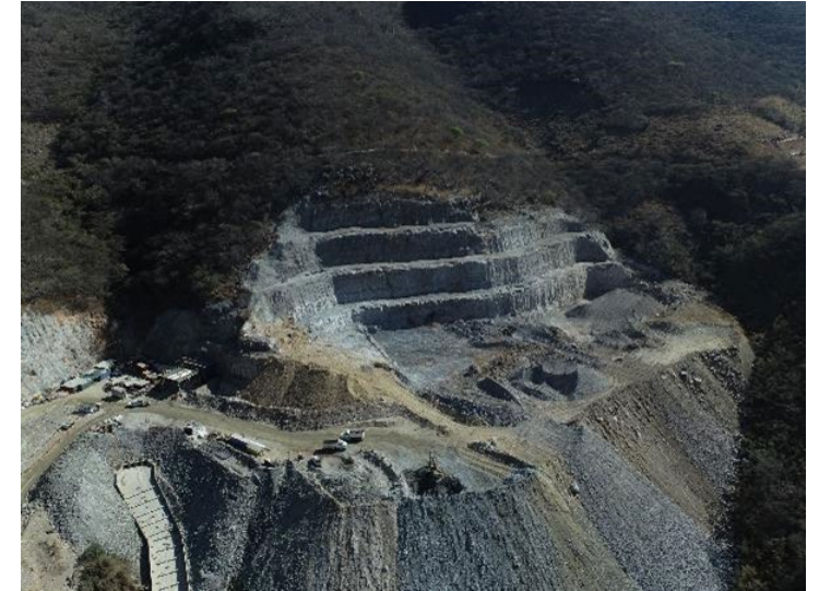
Paste plant pad preparation
