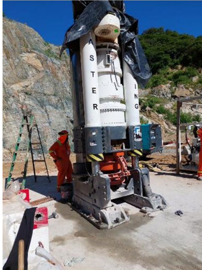
Setting up the raise bore machine
