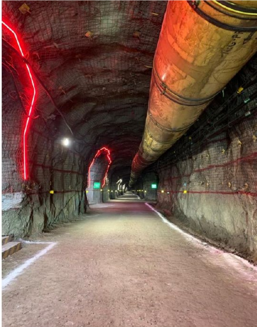
South Portal Lower tunnel
