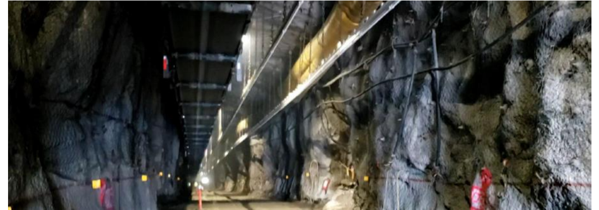
Total Guajes tunnel development of 450 m
