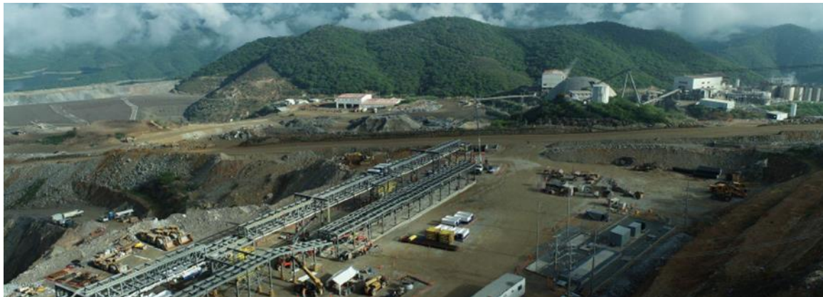
Overhead shot of loadout facility and plant
