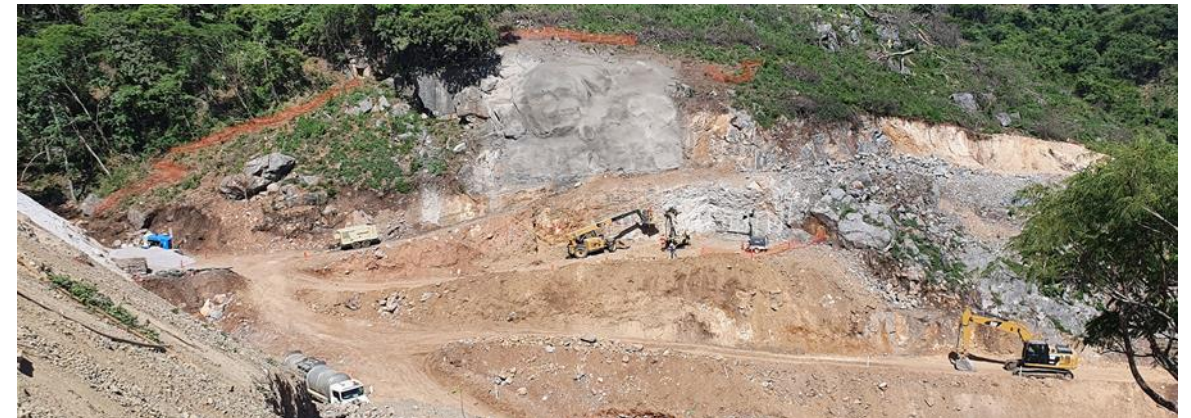
Prep of South Portal Upper well underway
