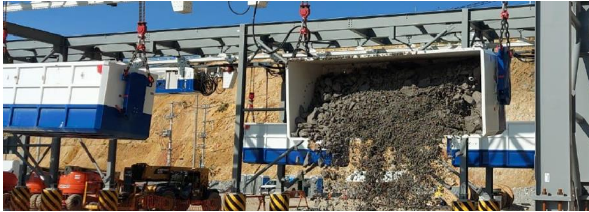
Monorail-based haulage for waste rock
