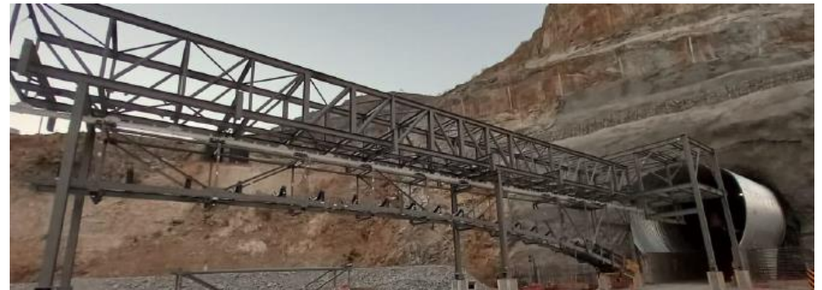
Installation of bridge conveyor
