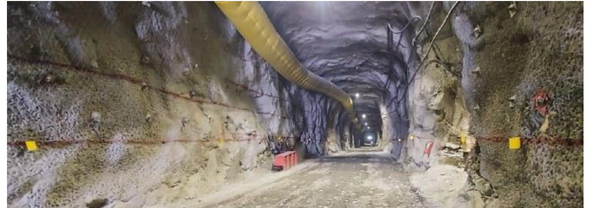
Guajes tunnel advanced ~300 metres
