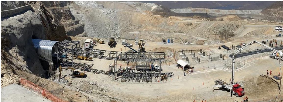
Steel infrastructure for monorail load-out
