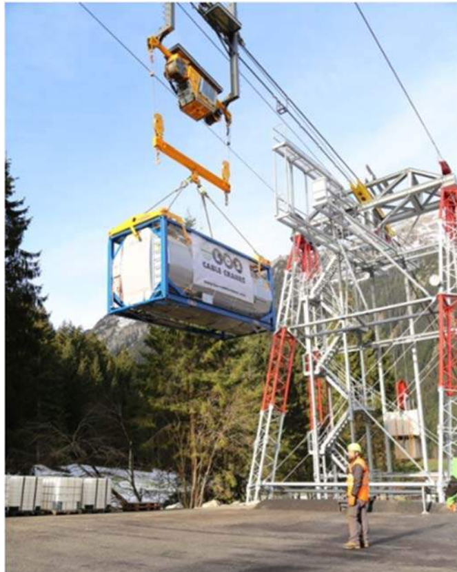
Figure 24-17: Ropeway Elevated Cable Crane System (Courtesy of LCS)
