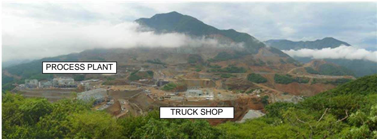
Figure Source: M3 Engineering, 2015. Photograph looks southeast. (Mine Infrastructure in foreground and Guajes pit behind.)
