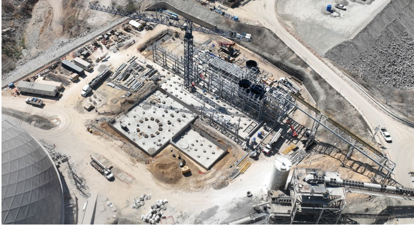
Surface construction at flotation circuit
