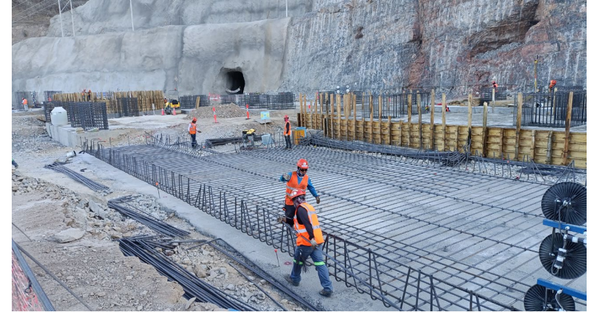
Concrete work for paste plant
