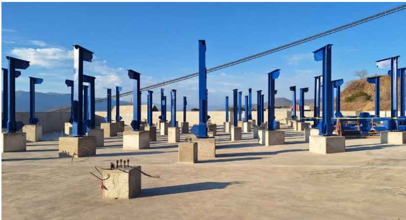
Steel erection at Guajes thickener
