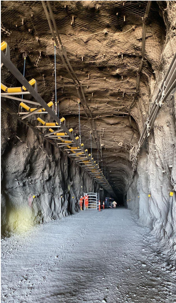
Conveyor table installation
