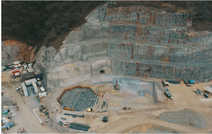
Concrete work in the paste plant thickener area
