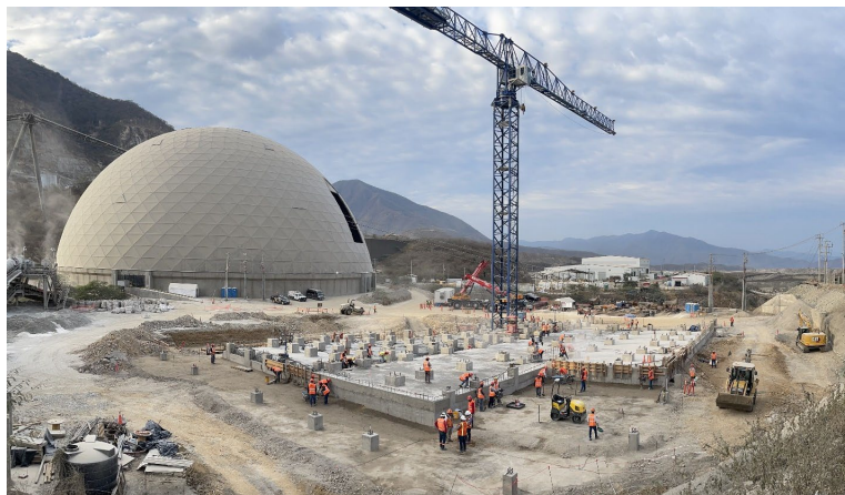
Concrete works at the flotation plant
