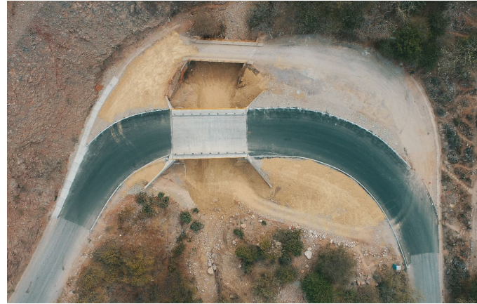
Mazapa bypass road and bridge are now complete
