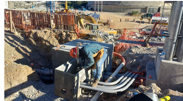
Installation of communication and electrical conduits
