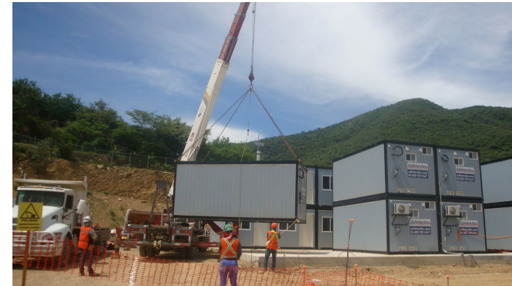
Installation of dormitory modules at contractor camp
