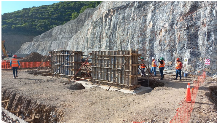
Foundation and electrical work for back-up generator stations
